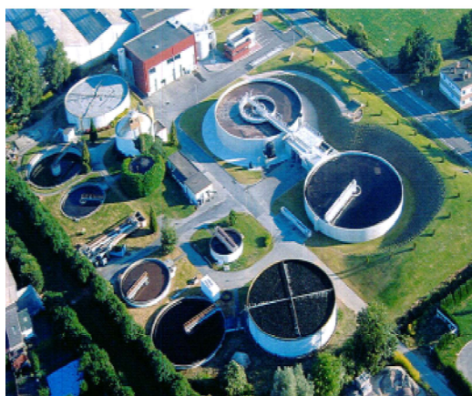
STATION D'EPURATION - HAZEBROUCK
