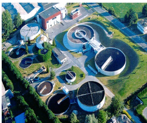
STATION D'EPURATION - HAZEBROUCK
